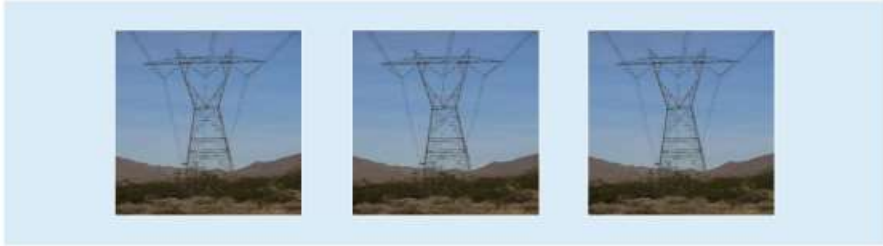
6 - 345 kV Single Circuits
