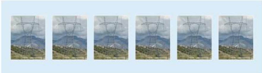
6 - 345 kV Single Circuits
