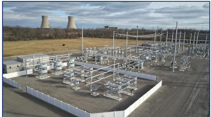
Phase II of the project involved the installation of a new 150 MVAR Static Var Compensator (SVC) at Toll Road Station, the first SVC installation in ITC's Michigan systems. SVCs provide an operational tool to ensure voltage stability for a diverse set of system conditions. This phase of the project was completed in December 2018. The Fermi-Vital 120 kV line was cut into the station in February 2019 following the SVC installation.
