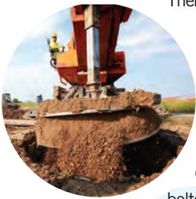
There will be 149 poles and towers in Tuscola County. Once the right-of-way is prepared, crews drill the foundations with large augers, lower the bolt cages and pour concrete. The foundations range from six to 12 feet in diameter and 25 to 60 feet deep.
