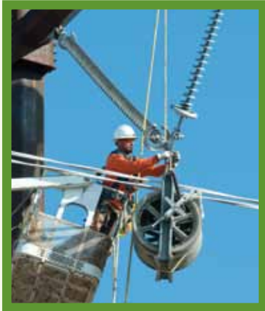
ITC contractor works to string wire on a new monopole.
