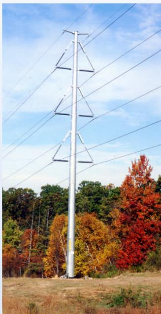
*ITC will replace older wood structures with new steel monopoles similar to the one shown here.*
