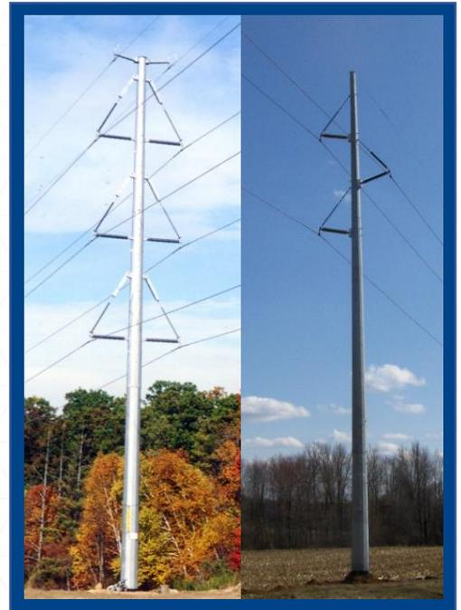
The new Long Rapids transmission line towers will be similar to the ones shown here. On the left is a double-circuit tower, and on the right is a single-circuit tower.
