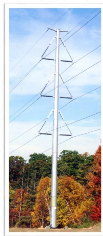
The new Bard Road – Warren double-circuit monopoles will be similar to the one shown here.
